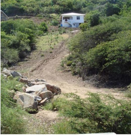
**Figure 9. Erosion (channelized within road cut) from house construction**
